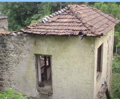
Micro-Hydro Plant in Vevchani
